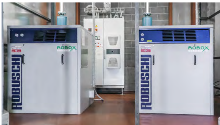
ROBOX screw installed at Barilla Plant in Parma
