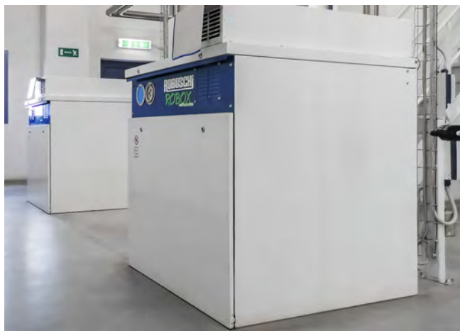
ROBOX screw installed at Barilla Plant in Parma
